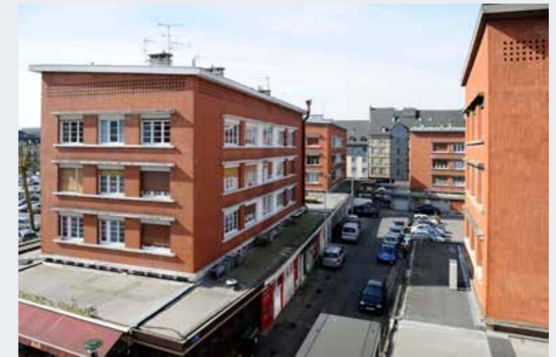
Lisieux, reconstructed center Architect in Chief: Robert Camelot ©Patrice Gourbin
