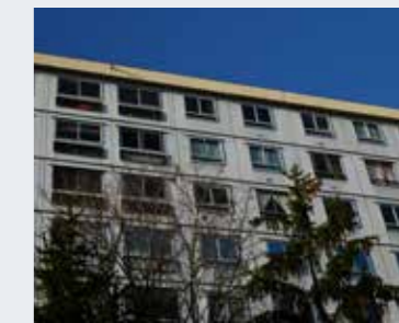
The Prouvé panels, south facade.
