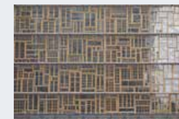
Facade of the European Council in Brussels, Belgium, with recycled chassis-frame base, 2016 Architect: Philippe Samyn © Pierre Belli-Riz
