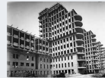
Beaujon Hospital during construction. APHP Archives (1934)
