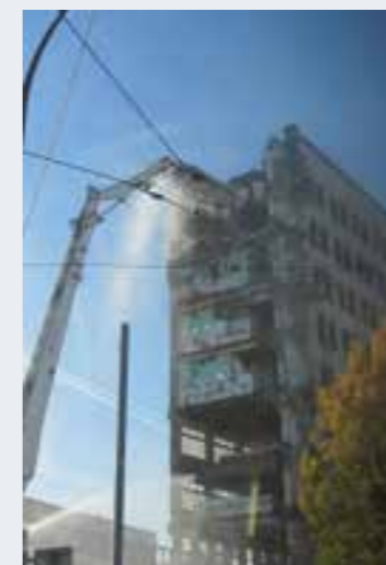
Demolition of a building in Grenoble, 2006 © Pierre Belli-Riz
